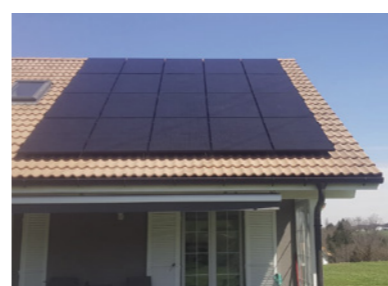
49 m 2 – 9.6 kWc 1695 Villarsel-le-Gibloux
